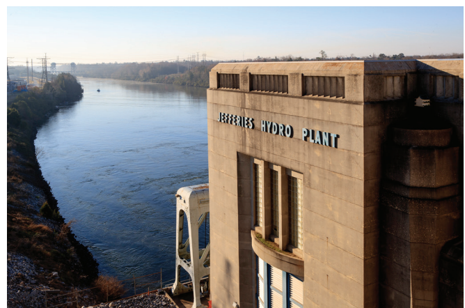
Jefferies Hydroelectric Generating Station
